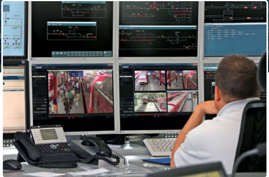
The control room has everything in view
