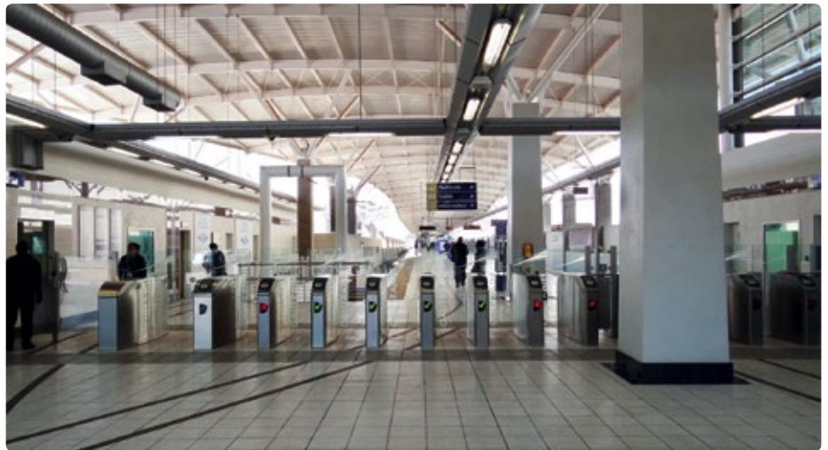
Discreet but all-seeing dome cameras at a typical station
