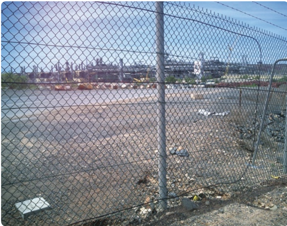
Secure Fence can pinpoint the location of intrusions to within 25 m anywhere along the fence, requiring no power or electronics.
