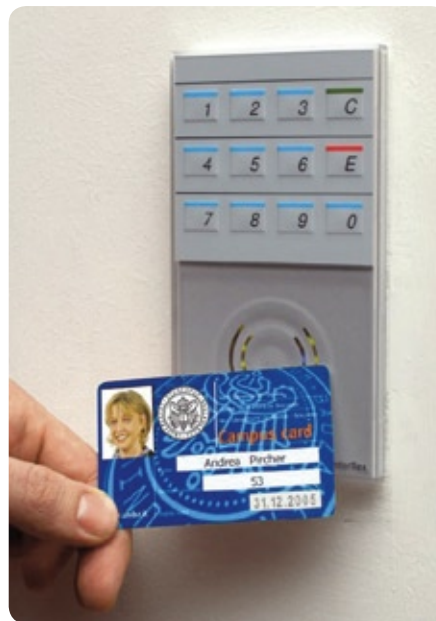
Access Control for a server room
