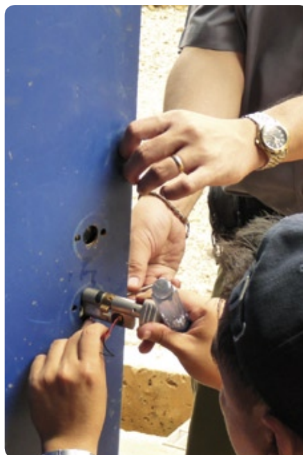
Staff from Thai security experts Skulthai installed the BlueChip locking cylinders.
