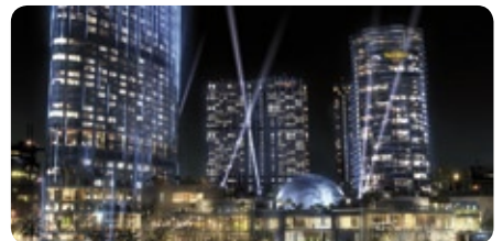
A City of Dreams Video Security Technology for the new „City of Dreams“ in Macau
