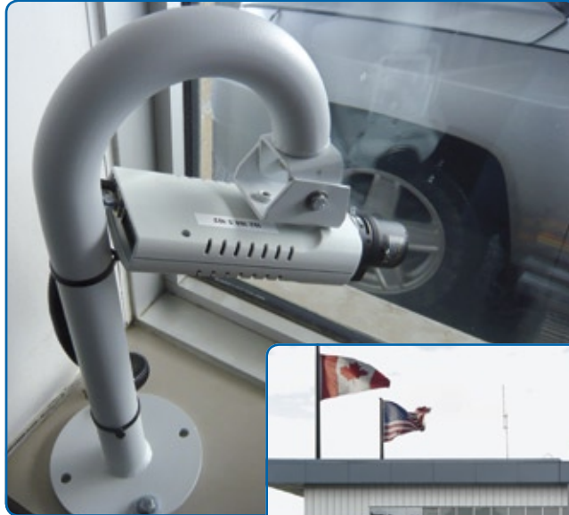
IndigoVision's HD Fixed IP cameras monitor traffic passing through each check-point.
