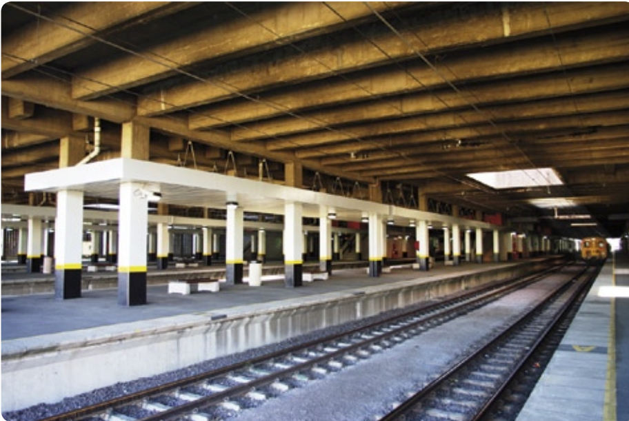
Durban Metro Rail: on of the station platforms
