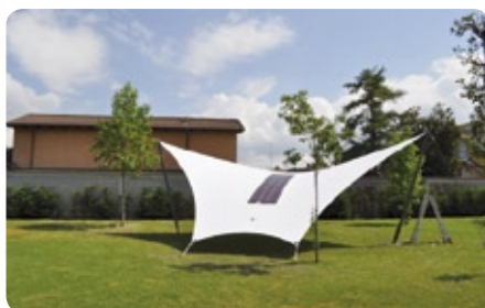
Fig. 1b: Demonstration of integrated solar cells in a textile membrane (Context)
