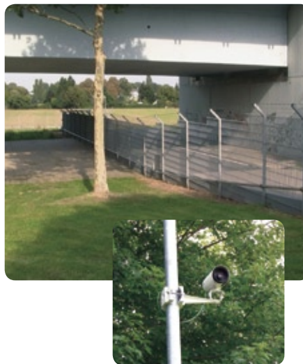
These thermal imaging cameras from FLIR monitor one of the flood-threatened areas. They need no lighting to be effective and due to their long range capacity they can cover the entire area from a safe distance.
