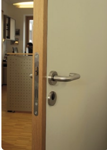
Almost 700 doors in the main building and the hospital surgery department have already been equipped with intelligent EZK door handle sets, a product jointly developed by FSB and Winkhaus
