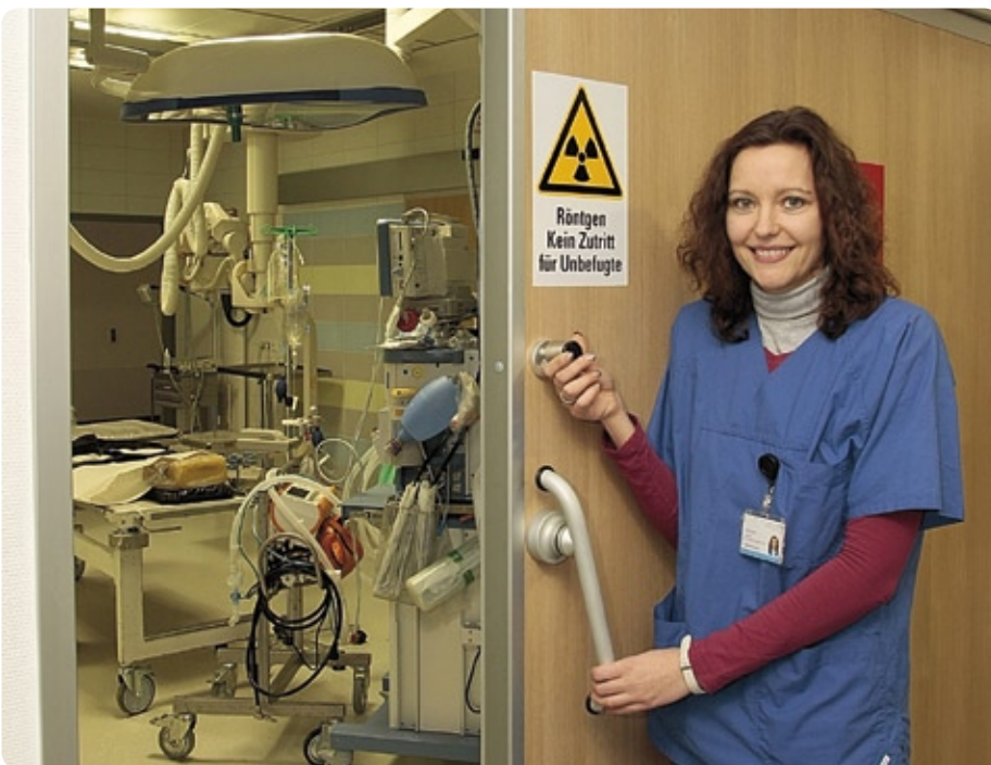
Hospital employees use Winkhaus electronic double knob cylinders to open sliding doors. Employees' cards are identified as identity media by the contactless system when they are held against the cylinder.
