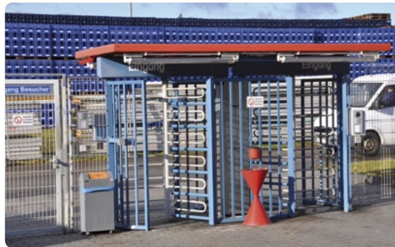
Gerolsteiner uses Argus, Geutebruck's high speed pan & tilt camera to monitor the perimeter fence and the turnstile entrance as well as the public helicopter pad.
