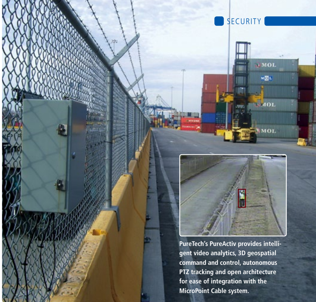
Southwest Microwave's MicroPointCable system pinpoints fence cut or climb attempt to within 3m, while ignoring environmental disturbances such as wind, rain or vehicle traffic.
