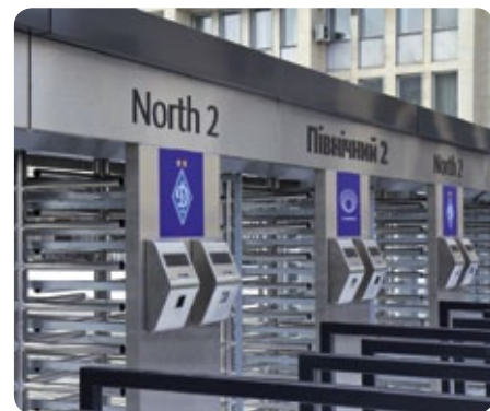
Full height turn-stiles with integrated ticket readers at the entrances
