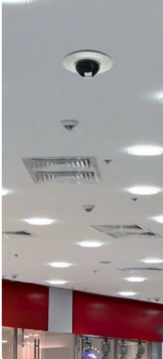
Suspended ceiling kits are used to flush-mount the IP dome cameras in the ceiling.
