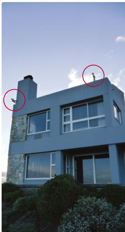
For aesthetic reasons some Flir Systems thermal imaging cameras are mounted on the house instead of a mast.
