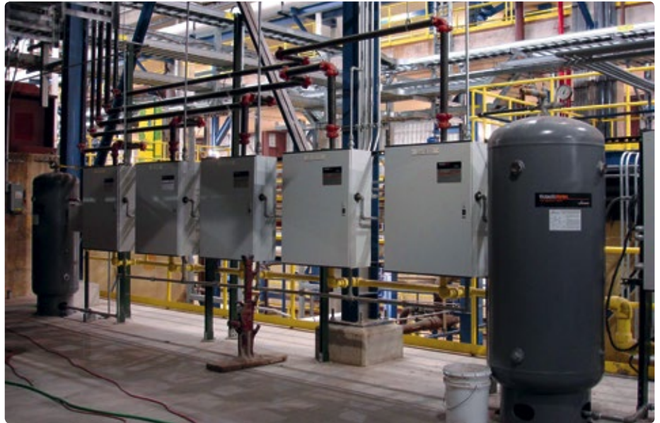
The Vortex 1000 and 1500 fire suppression systems for industrial applications
