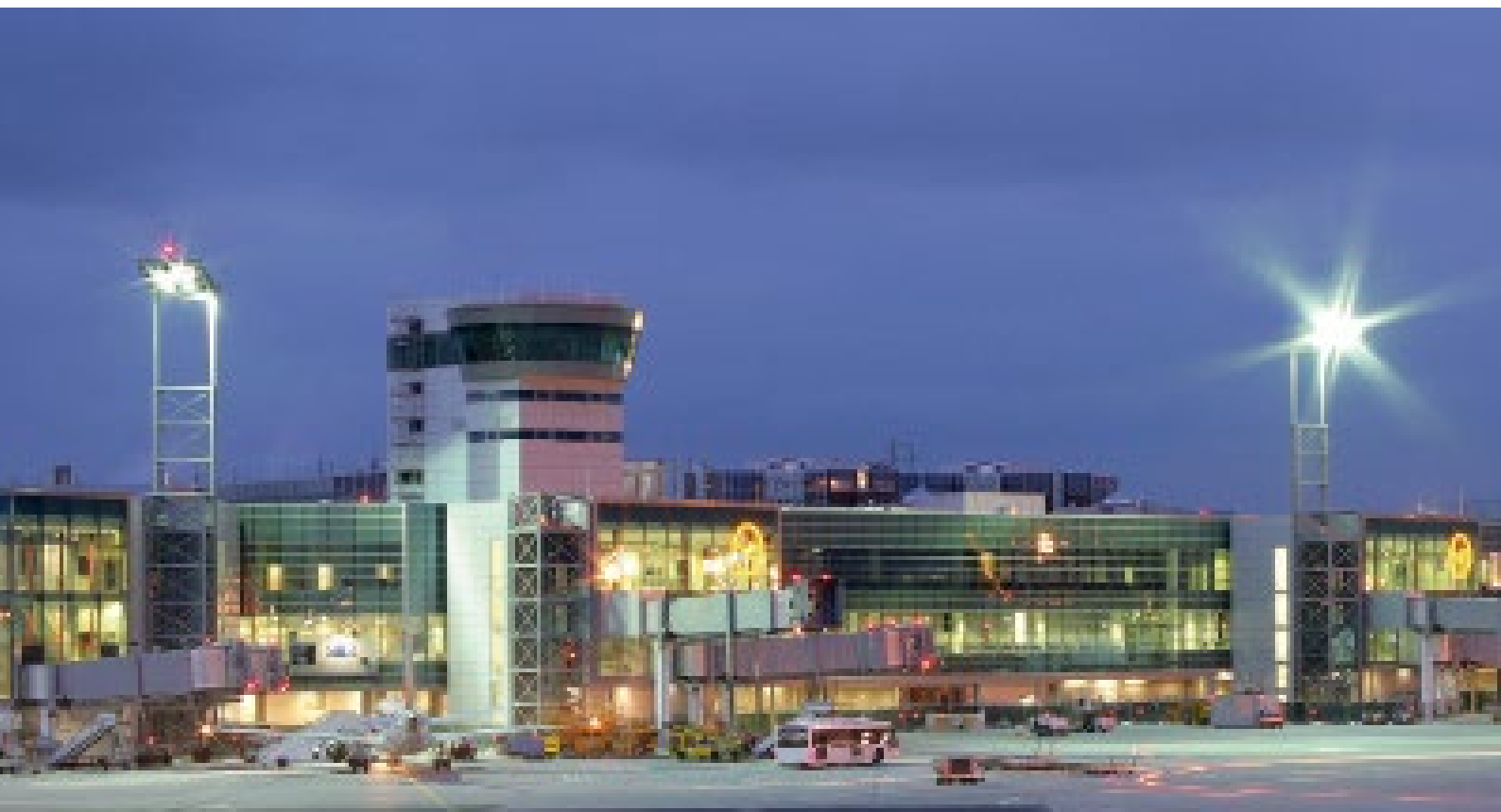
The movement area of the Frankfurt airport at night
