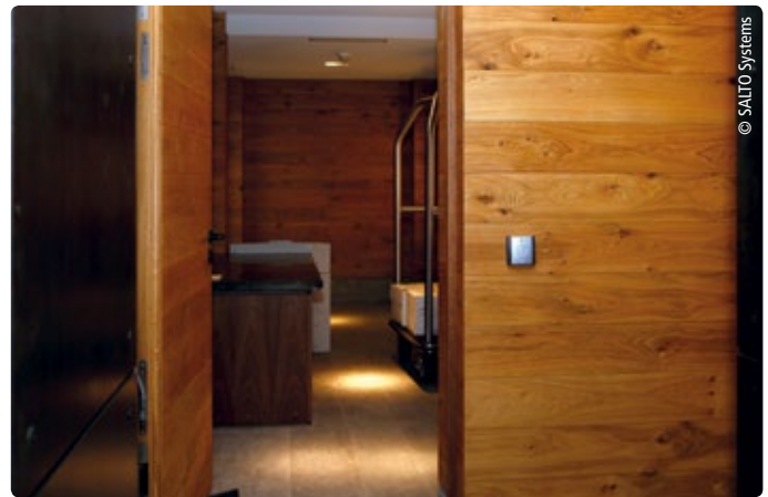
The locker room is secured by a XS4 Original wall reader
