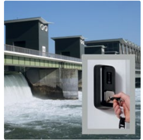
High security for critical installations
