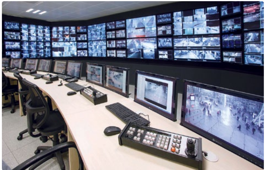
Airport security staff can view the airport's CCTV, access control, fire safety systems and also intrusion systems from the central control room.
