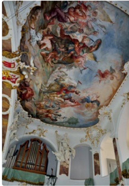
The ASD pipework can be made practically invisible, therefore it can be also used for artistically decorated ceilings.
