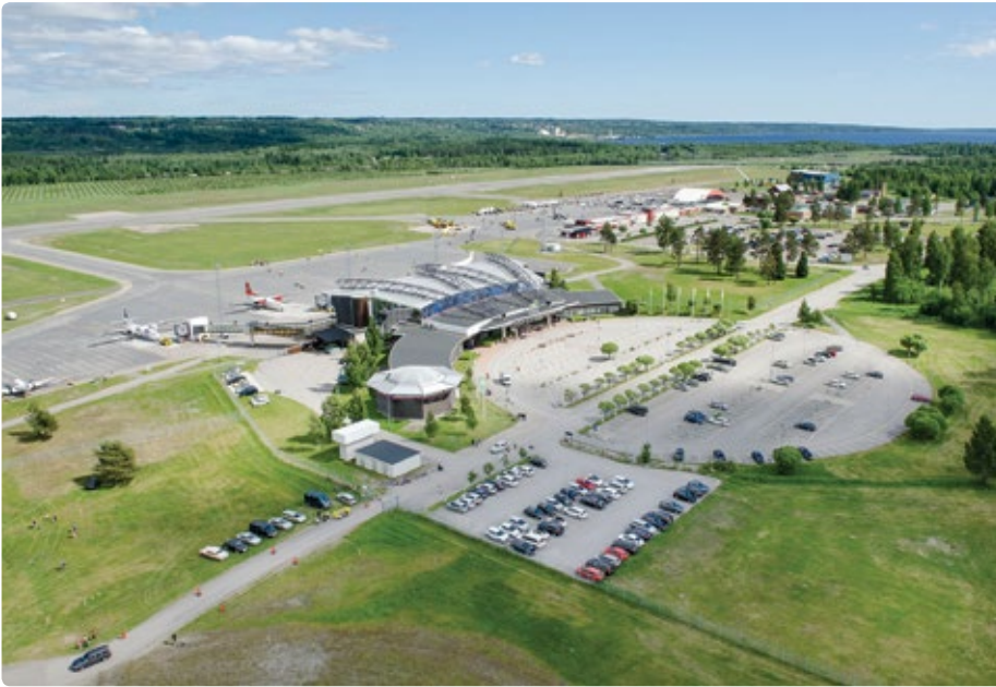
Security Center offers Sundsvall Airport a highly-advanced security solution meeting EU regulations
