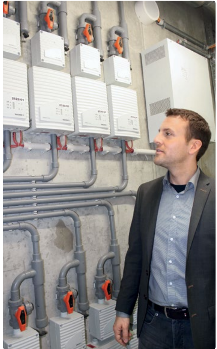
Dennis Just, Technical Manager at Hamburg’s Elbe Philharmonic Hall with some of Wagner’s air sampling technology
