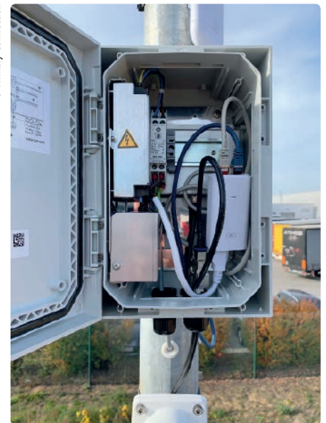
All-in-one solution for secure video surveillance. An outdoor network interface box with attached day/night camera and WLAN bridge
