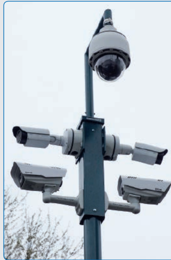
High resolution cameras, Systems using AI and thermal cameras secure the data centers
