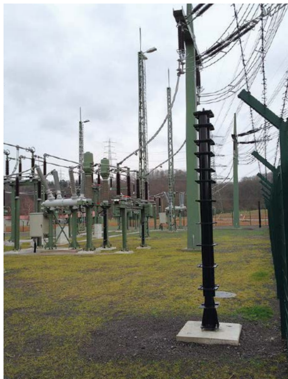
Communication occurs through a dynamic radio mesh network (through proprietary protocol) to and from all Solaris columns that transmit alarm information reliably and efficiently
