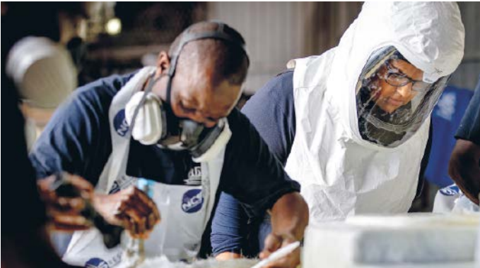
Maxwell Jara applies fiberglass mats and resin layer by layer. He is wearing a Dräger X-plore 3500 half mask with combination filters.
