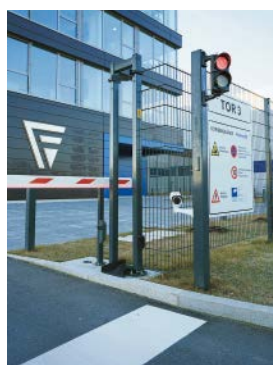
Access management via number plate recognition with Dallmeier box cameras and ANPR solution
