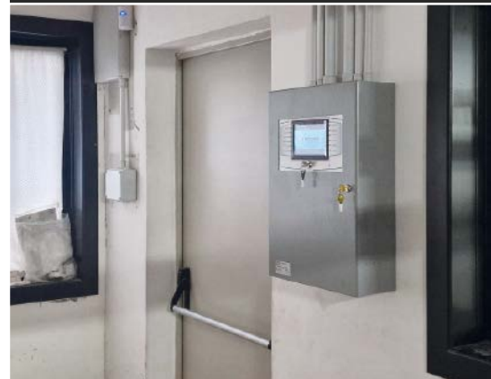
Fire doors are integrated into the Latitude panel network, enabling real-time door status monitoring and ensuring rapid, panel-coordinated compartmentalisation during an alarm event
