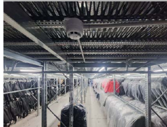
Hochiki ESP intelligent sensors paired with YBO-BSB2 base sounder beacons provide unified audio-visual signalling throughout the open warehouse, ensuring clear alerts even in high-noise operational areas
