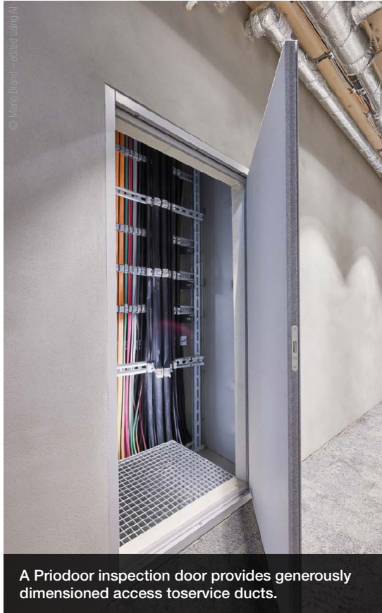
The Priodoor RTX inspection door provides fire-resistant partitioning of cable ducts in data centers.
